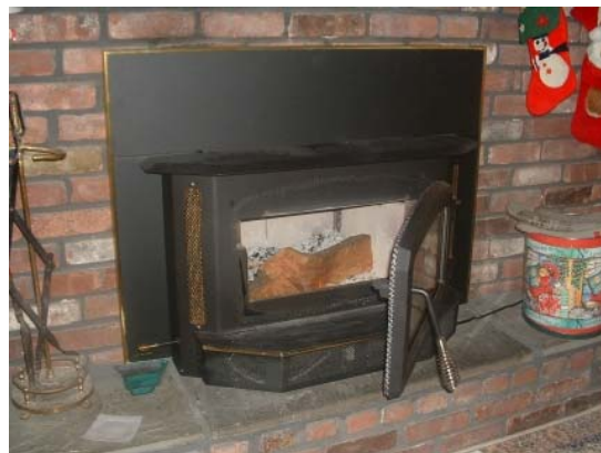
Wood burning insert installed in an already existing fireplace.
